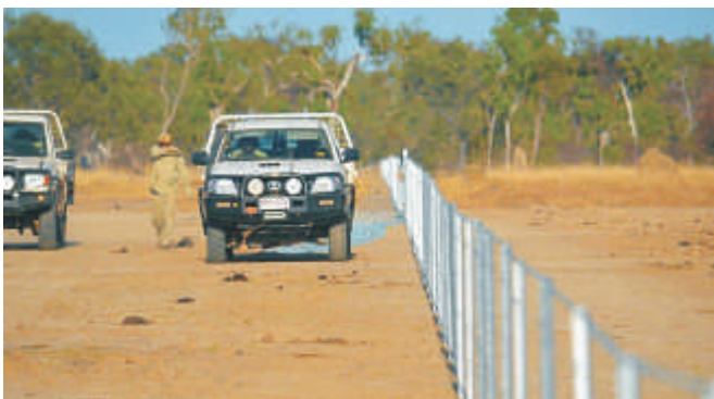
Exclusion fence work at Lotus Lagoon, Delta Downs Station, extending a total of 7km and protecting approximately 200ha of wetland
